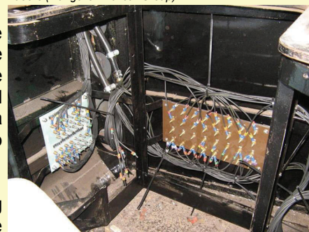
Cab rewiring in 56097 (Llangollen Railcar Group)
